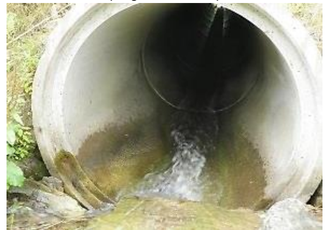
Figure 3-80: Example of a crossings with an inlet drop. (Image credit: NAACC)
