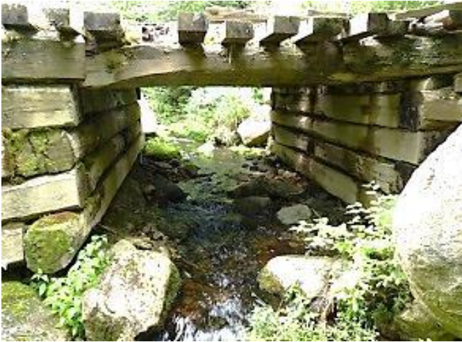
Figure 3-42: Example of a bridge with abutments. (Image credit: NAACC)
