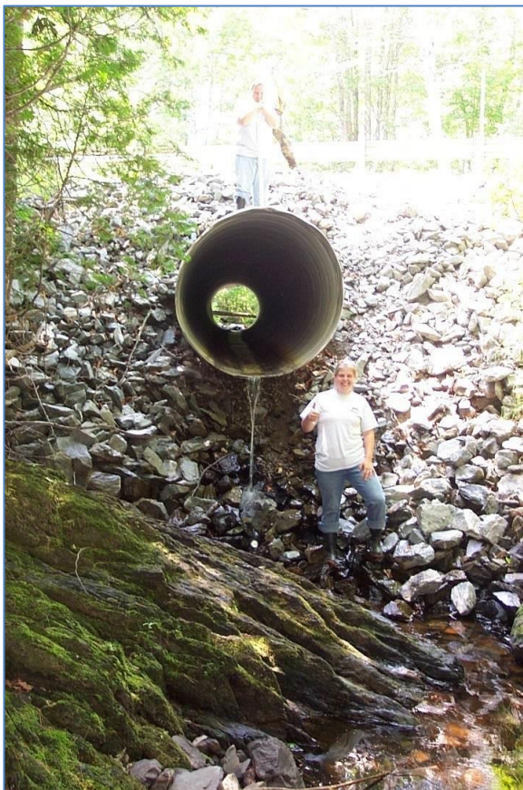
Figure D-7. An additional example of a good photograph. This photo shows adequate context around the structure, including a field data collector in a safe position near the structure for scale, the roadway and bank above the culvert, and the stream downstream of the culvert (including the full width of the culvert). Note that the photograph is overexposed, reducing the available contextual information about the road at the top of the photograph. (Image credit: NAACC)
