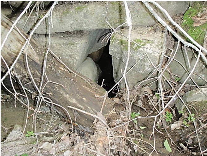
Figure 3-95: An example of a crossing structure with multiple barriers. The culvert is deformed by displaced stones, blocked by debris, and dry. (Image credit: NAACC)
