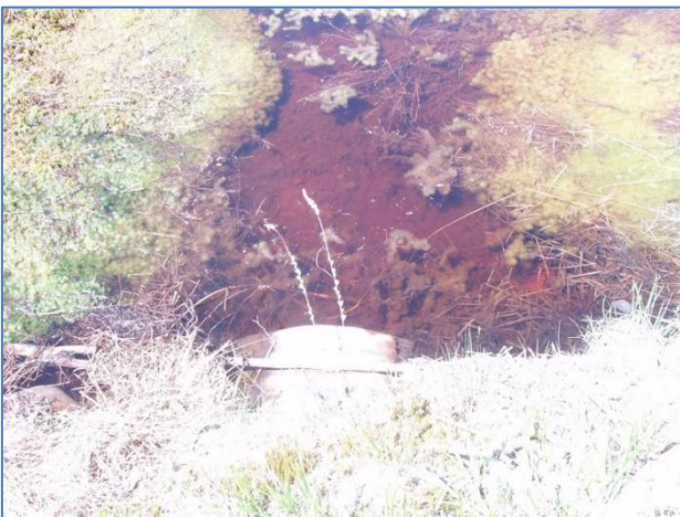
Figure D-11. An example of a downstream photograph that shows very little context of the crossing. Note that the photo is also overexposed, which limits the information available in the photo. This photo could be improved by adjusting the angle of the photo to capture more of the downstream channel and adjusting the settings to avoid overexposure (Image credit: NAACC).
