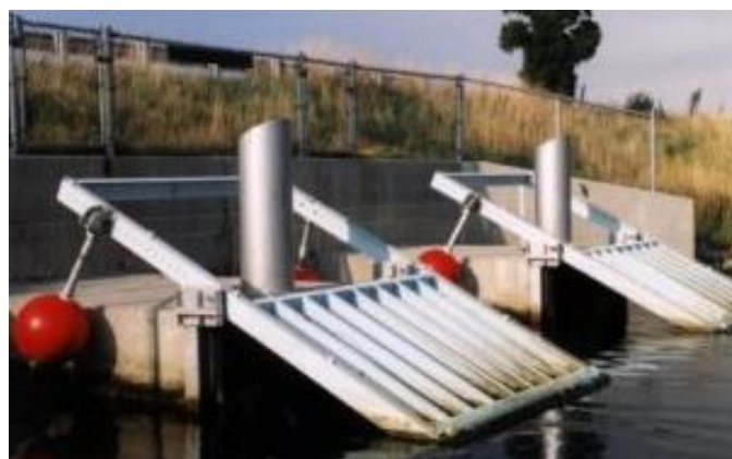
Figure 3-24: Self-regulating tide gate. (Image credit: URI)
