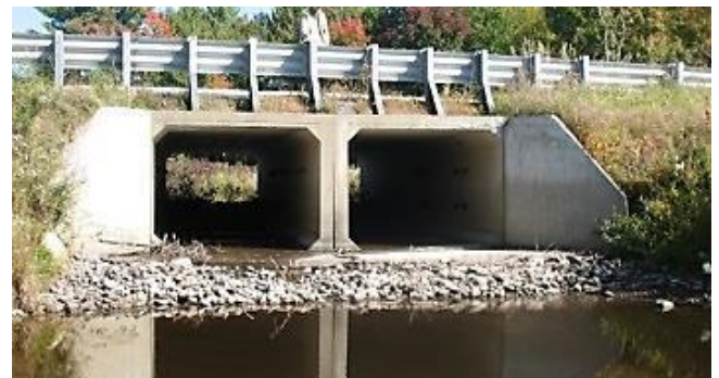
Figure 3-2: Example of a road-stream crossing consisting of multiple box culverts. (Image credit: NAACC)
