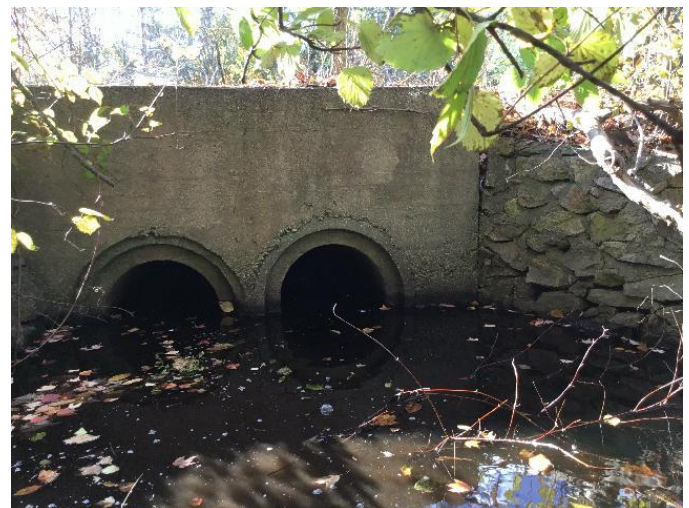
Figure 3-67: Example of crossings with headwalls with a chamfered or beveled edge.
