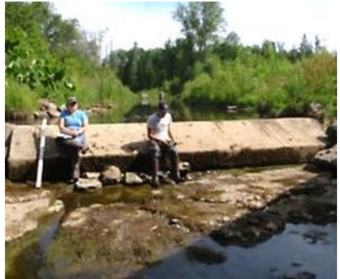
Figure 3-93: A dam with no free fall acting as a physical barrier at a crossing. This physical barrier would be classified as "Other." (Image credit: NAACC)
