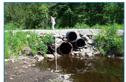
Figure D-2. Examples of good outlet photographs that are taken far enough away from the structure so that the entire structure is visible and the surrounding fill, armoring, and streambanks are captured.
