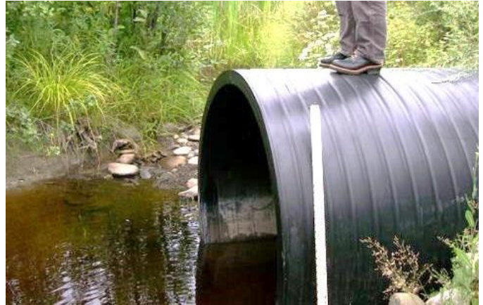
Figure 3-31: Material – Smooth plastic. (Image credit: NAACC)
