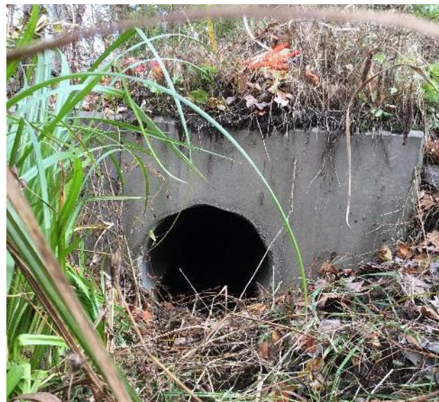
Figure 3-65: Examples of crossings with headwalls with square edges. (Image credit: NAACC)
