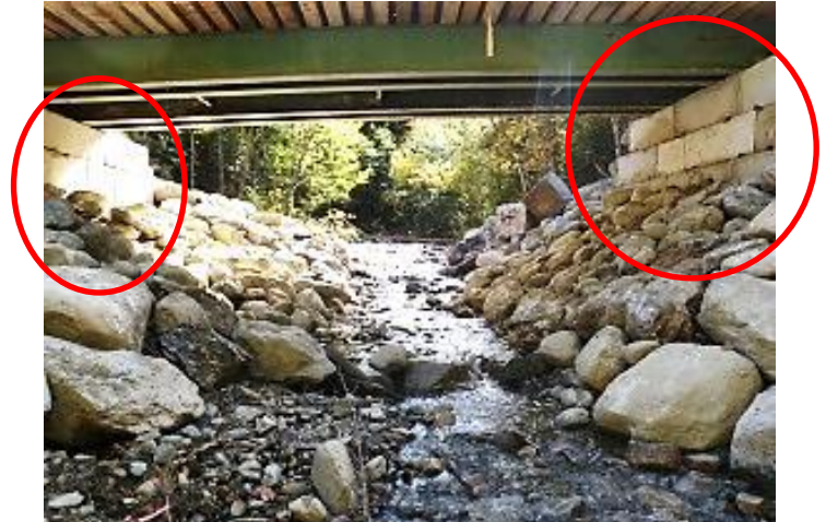
Figure 3-44: Examples of bridges with abutments and side slopes. The abutments are indicated by the red circles. (Image credit: NAACC)
