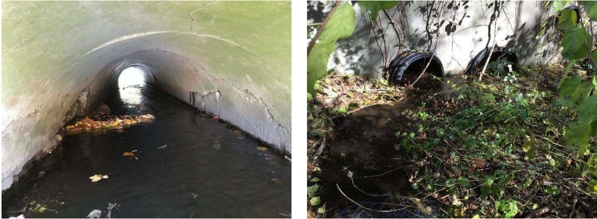
Figure 24. Poor Barrel Condition of xy41834977144282 on Pleasant Valley Parkway in Providence (unnamed tributary to Woonasquatucket River) (left) and level of blockage of xy41888657151262 on Farnum Pike in Smithfield (unnamed tributary to Georgiaville Pond)(right).
