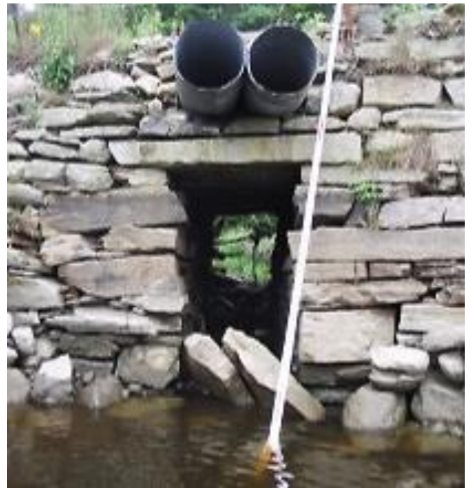
Figure 3-101: An example of multiple structures at a crossing, each with a physical barrier. The lower, rectangular stone culvert is blocked by fallen stones. The two metal culverts above are dry. (Image credit: NAACC)
