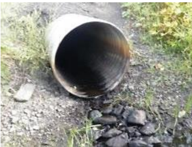
Figure 3-48: Examples of crossings with an outlet apron that is not extensive. (Image credit: NAACC)
