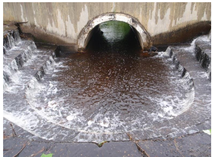
Figure 3-88: Free falls acting as physical barriers. (Image credit: NAACC)
