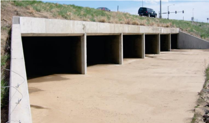
Figure 3-70: Example of a headwall with beveled or chamfered edge and wingwalls (Image credit: Schall et al., 2012).
