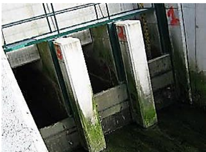
Figure 3-21: Stop log tide gate. (Image credit: NAACC)
