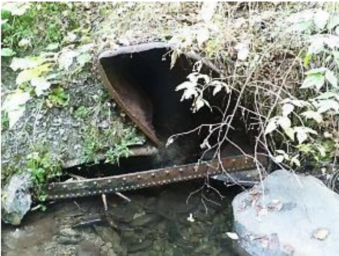
Figure 3-99: An example of a crossing structure with multiple barriers: the culvert is deformed, blocked by debris, and dry. (Image credit: NAACC)
