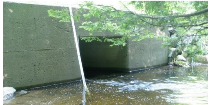
Figure 3-66: Example of a crossing with headwall with square edges. (Image credit: NAACC)
