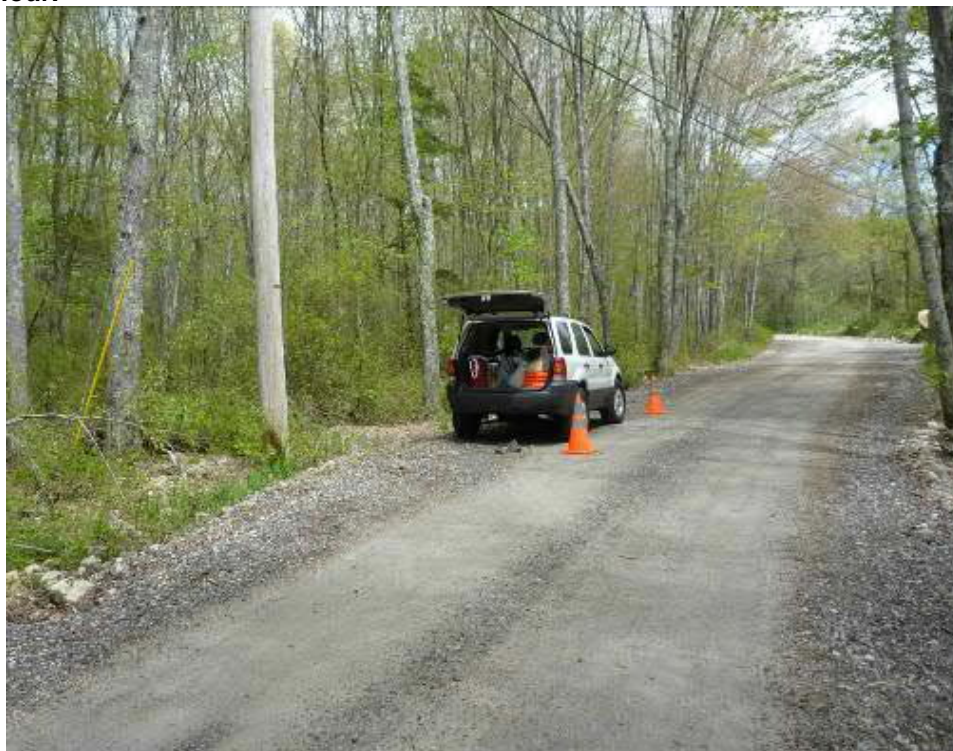
Figure 2. Cones set up on relatively high speed state route. Travel lanes are not blocked, and work will be less than one hour.
