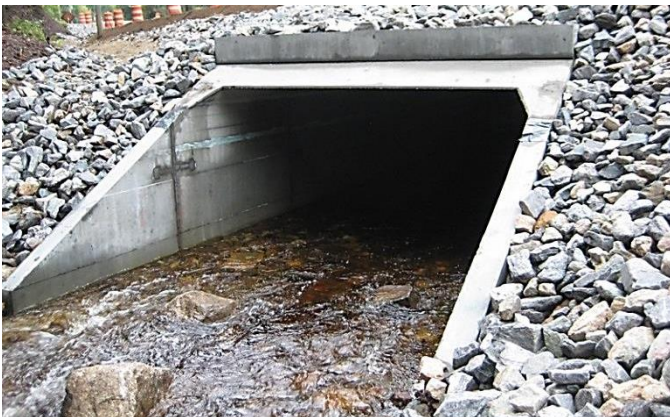
Figure 3-70: Example of a headwall with beveled or chamfered edge and wingwalls (Image credit: Schall et al., 2012).
