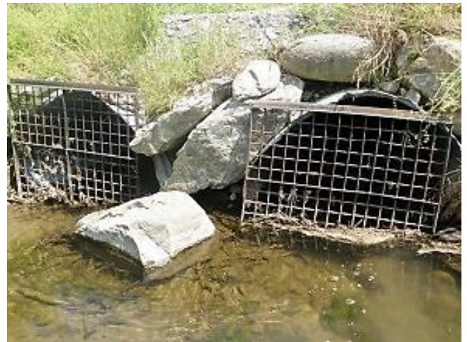
Figure 3-90: Fencing acting as physical barriers. (Image credit: NAACC)
