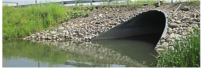
Figure 3-72: Example of a crossing with inlet that is mitered to the slope. (Image credit: NAACC)
