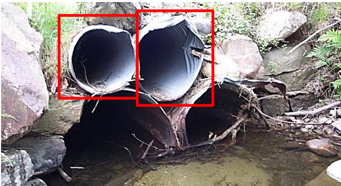
Figure 3-91: Dry culverts (indicated by the red boxes) acting as physical barriers. (Image credit: NAACC)
