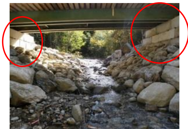
Figure 3-62: Examples of bridges with side slopes and abutments. The red circles indicate the abutments. (Image credit: NAACC)
