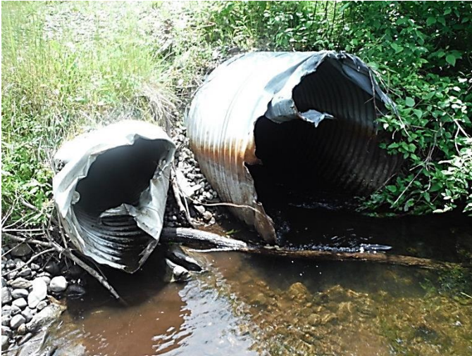
Figure 3-94: An example of a structure with multiple barriers. The culvert on the left is deformed and dry. (Image credit: NAACC)
