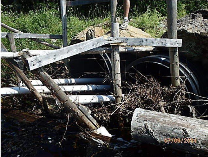
Figure 3-98: An example of a crossing structure with multiple barriers: the culvert is blocked by debris and fencing. (Image credit: NAACC)
