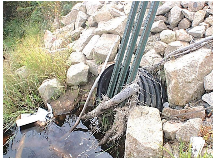
Figure 3-97: An example of a structure with multiple barriers. The culvert on the left is deformed (bent upward) and blocked by debris. (Image credit: NAACC)
