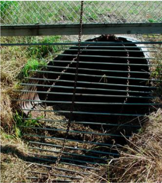
Figure 3-89: Fencing acting as physical barriers. (Image credit: USDA)
