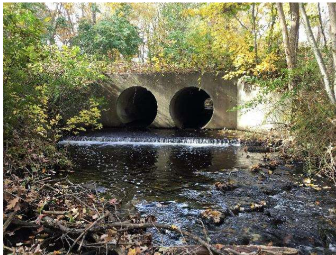
Figure 20. Outlet armoring and outlet drop associated with xy41873187150300 on Dean Street in Smithfield (Hawkins Brook).
