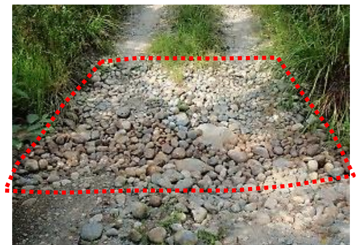
Figure 3-45: Examples of fords. (Image credit: NAACC)
