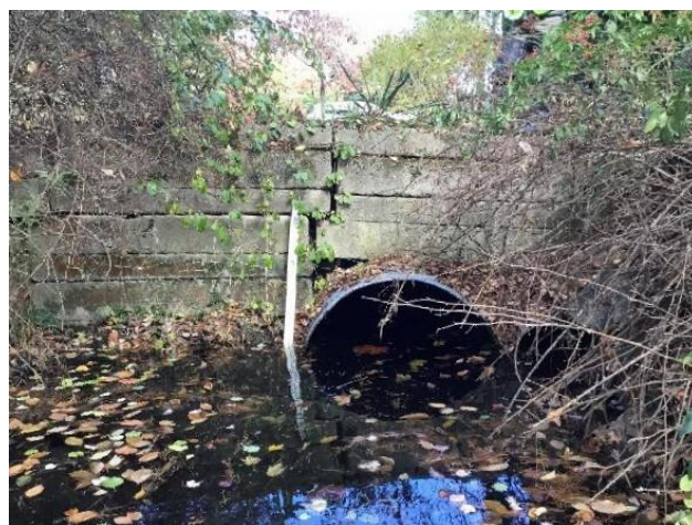
Figure 3-54: Example of a culverts with outlet at stream grade. (Image credit: NAACC)
