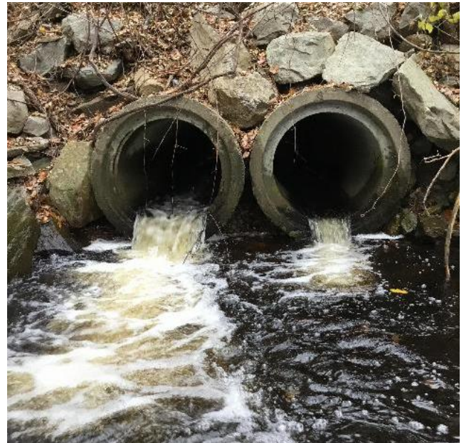
Figure 3-56: Examples of culverts with a free fall at the outlet. (Image credit: NAACC)
