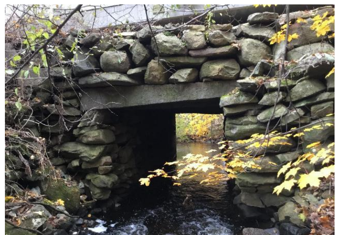
Figure 3-41: Examples of a box culvert and bridge with abutments. (Image credit: NAACC)
