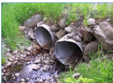
Figure D-1. Examples of good inlet photographs that show the surrounding context of the structure including the structure invert, the fill, and armoring.
