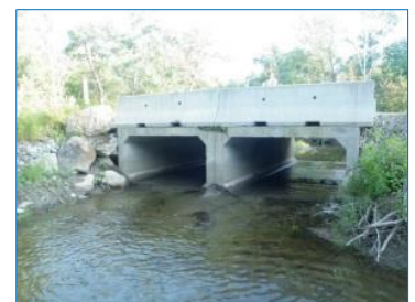
Figure D-1. Examples of good inlet photographs that show the surrounding context of the structure including the structure invert, the fill, and armoring.
