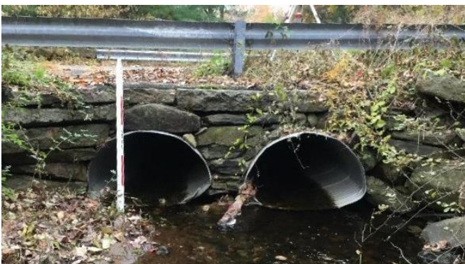
Figure 3-37: Outlet shape –Pipe arch/elliptical. (Image credit: NAACC)
