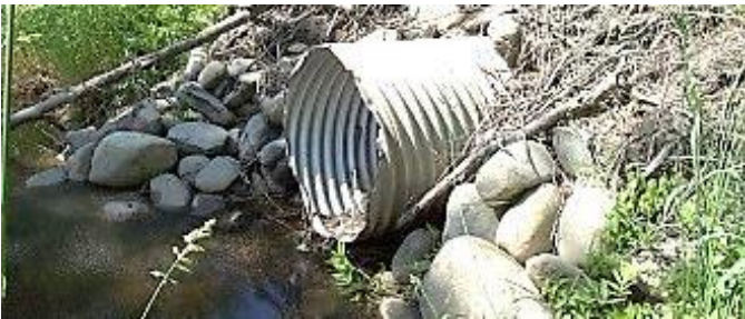
Figure 3-81: Examples of crossings with perched inlets. (Image credit: NAACC)
