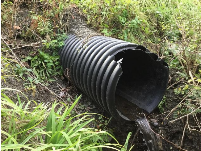
Figure 3-28: Material – Corrugated plastic (internal surface as well as external). (Image credit: NAACC)
