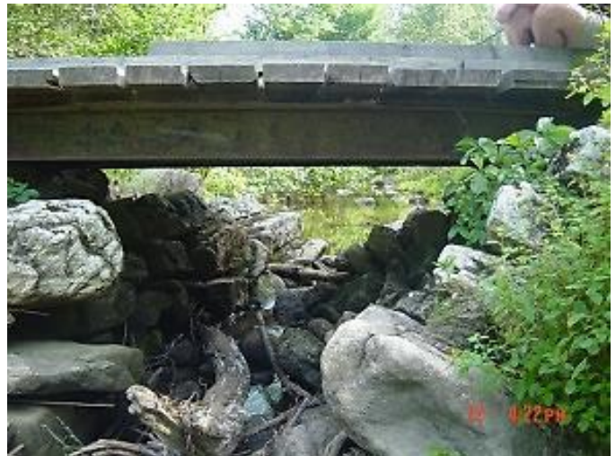
Figure 3-72: Example of a crossing with inlet that is mitered to the slope. (Image credit: NAACC)
