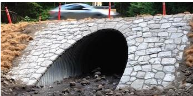
Figure 3-71: Examples of crossings with inlets that are mitered to the slope. (Image credit: NAACC, National Park Service)
