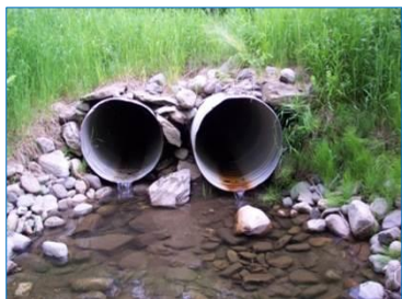
Figure D-2. Examples of good outlet photographs that are taken far enough away from the structure so that the entire structure is visible and the surrounding fill, armoring, and streambanks are captured.
