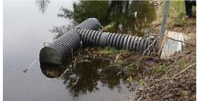
Figure 3-92: An anti-beaver attached to a crossing inlet acting as a physical barrier at a crossing. This physical barrier would be classified as "Other." (Image credit: NAACC)
