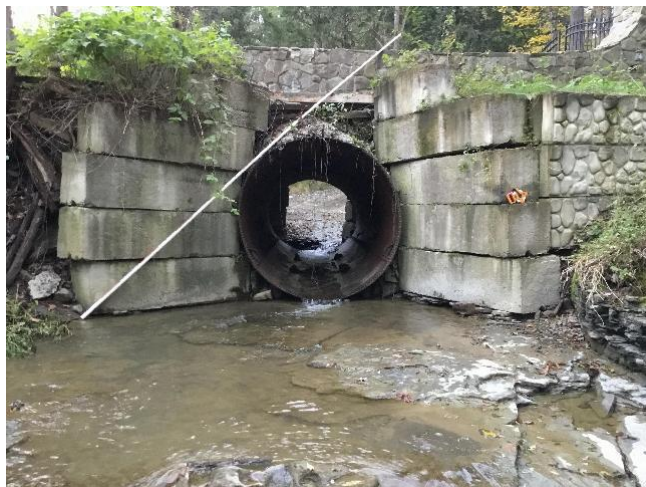
Figure 3-68: Examples of crossings with wingwalls. (Image credit: NAACC)
