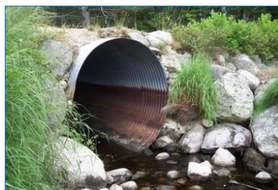
Figure D-1. Examples of good inlet photographs that show the surrounding context of the structure including the structure invert, the fill, and armoring.
