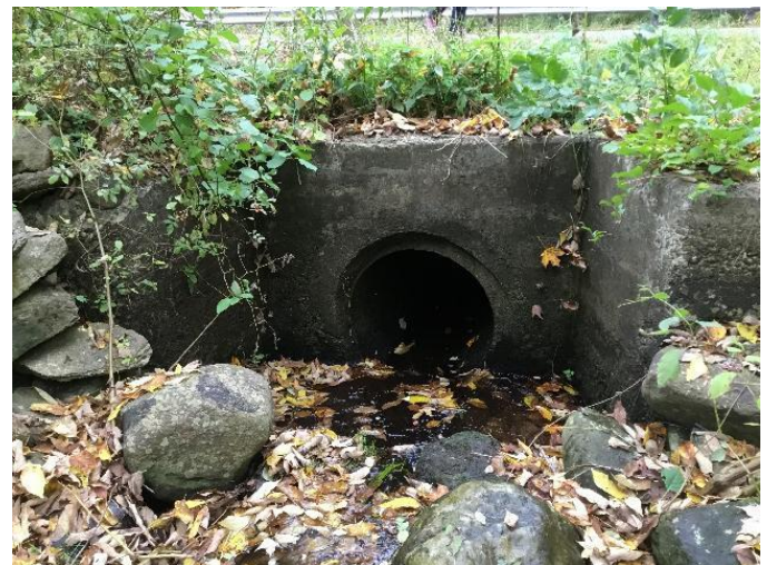
Figure 3-66: Example of a crossing with headwall with square edges. (Image credit: NAACC)
