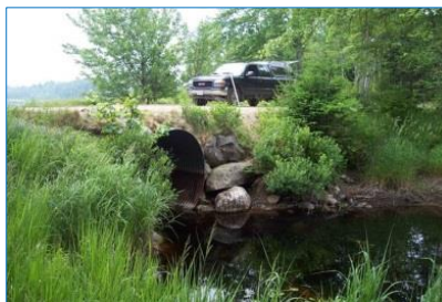
Figure D-2. Examples of good outlet photographs that are taken far enough away from the structure so that the entire structure is visible and the surrounding fill, armoring, and streambanks are captured.
