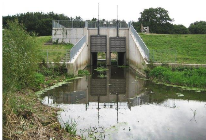
Figure 3-23: Sluice tide gate. (Image credit: Nigel Cox)
