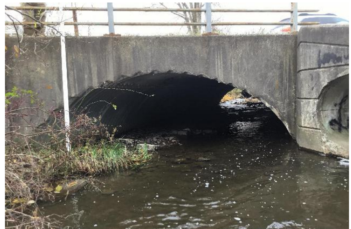
Figure 3-38: Outlet shape – Open-bottomed arch culvert and bridge. (Image credit: US Fish & Wildlife Service)
