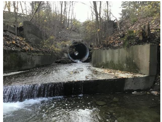
Figure 3-47: Examples of crossings with an extensive outlet apron. (Image Credit: NAACC and Fuss & O'Neill)
