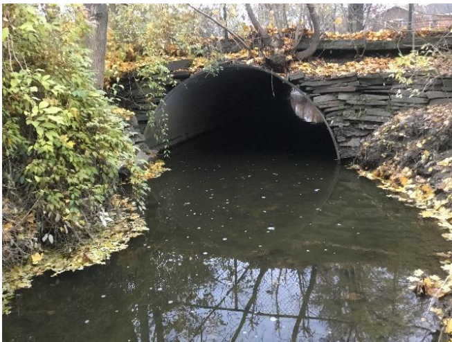
Figure 3-55: Examples of culverts with outlets at stream grade. (Image credit: NAACC)
