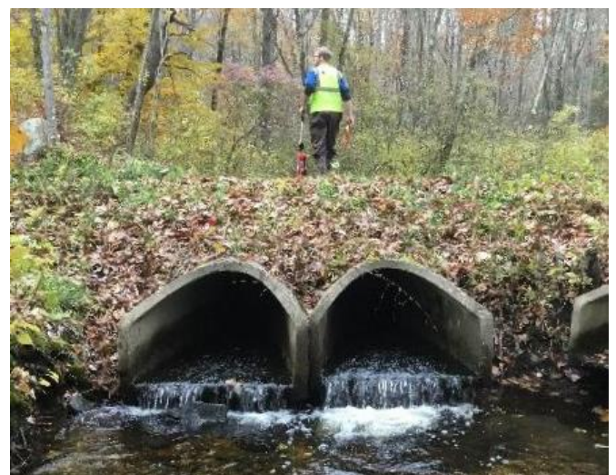
Figure 3-49: Examples of crossings with no outlet apron. (Image credit: NAACC)
