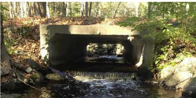
Figure 3-39: Outlet shape – Box culverts.
