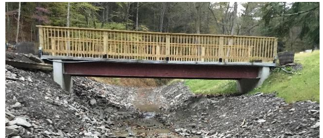
Figure 3-1: Example of a road-stream crossing consisting of a bridge with side slopes and abutments.
