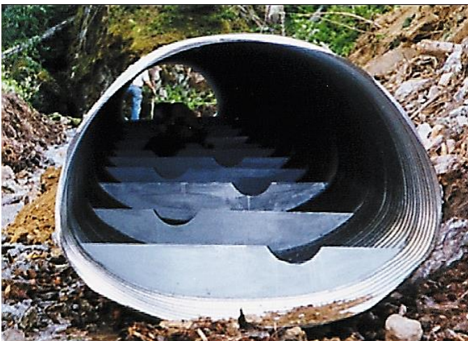
Figure 3-83: Examples of crossings with baffles and weirs. (Image credit: NAACC)
