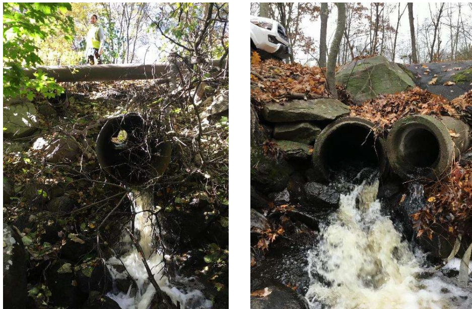
Figure 29. Outlet Drops associated with xy41848877150503 on Pine Hill Avenue in Johnston over Assapumpset Brook (left) and xy41890377149584 on Ridge Road in Smithfield over an unnamed tributary to the Woonasquatucket River (right)
