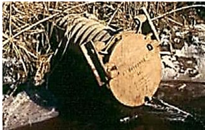
Figure 3-22: Flap tide gate. (Image credit: NAACC)
