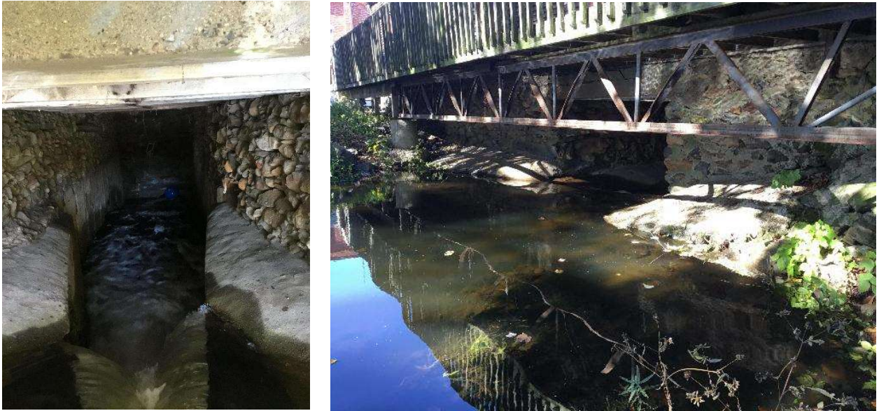
Figure 19. Inlet drop (left) and severe channel constriction (right) associated with xy41871207155179 on Putnam Pike in Smithfield, at the Slack Reservoir outflow.
