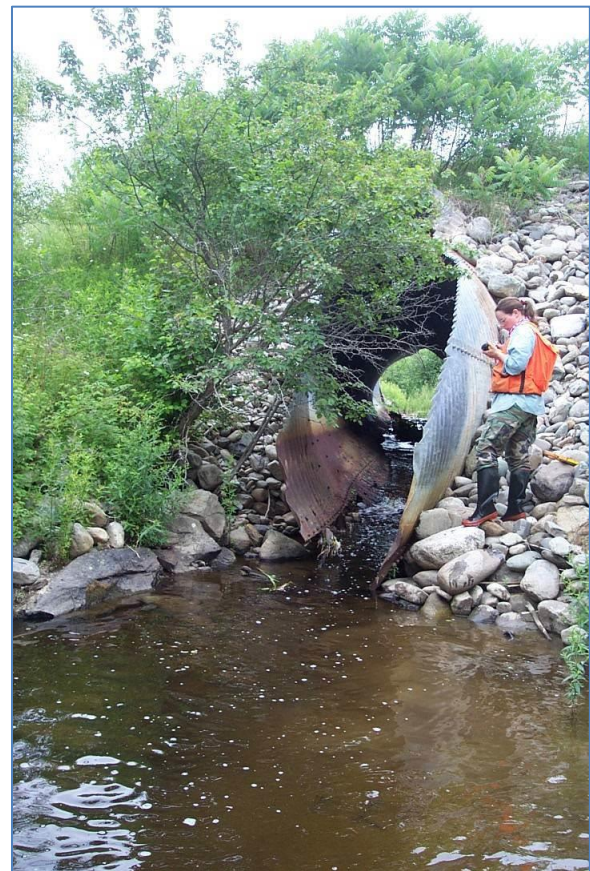
Figure D-8. An additional example of a good photograph. The photo shows the structure opening and surrounding armor, the roadway and bank above, and the stream outside of the structure (including the full width of the stream). The photograph also shows a Field Data Collector standing in a safe position near the structure, which provides a reference for the scale of the objects in the photograph (Image credit: NAACC)
