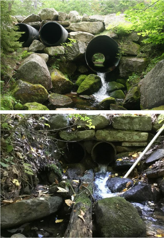
Figure 3-59: Examples of culverts with a free fall onto cascades at the outlet. (Image credit: U.S. Fish and Wildlife Service, NAACC)
