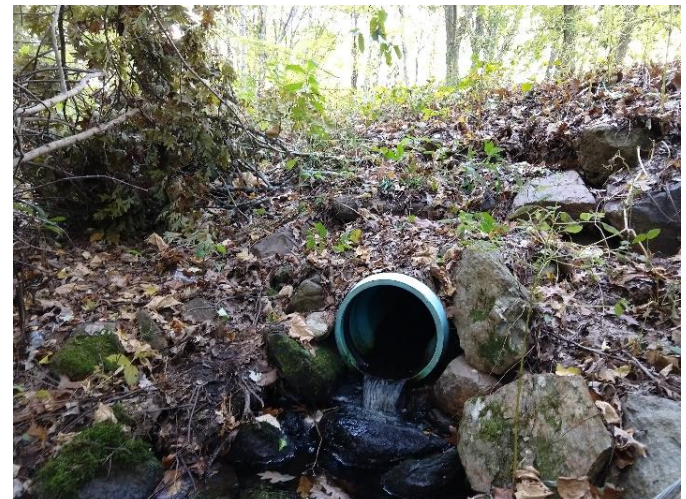
Figure 3-58: Examples of culverts with free falls onto cascades at the outlet. (Image credit: NAACC)
