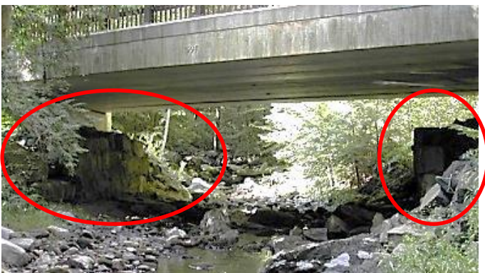
Figure 3-43: Examples of bridges with abutments and side slopes. The abutments are indicated by the red circles. (Image credit: NAACC)
