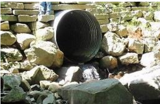
Figure 3-57: Examples of culverts with cascades at the outlet. (Image credit: NAACC)
