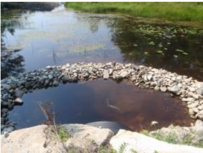
Figure 3-85: Stone acting as a physical barrier. (Image credit: NAACC)
