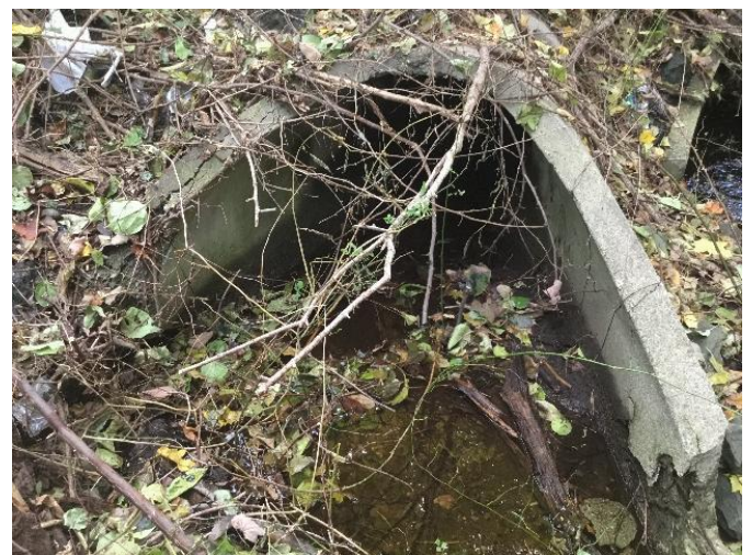
Figure 3-86: Debris acting as physical barriers. (Image credit: NAACC)
