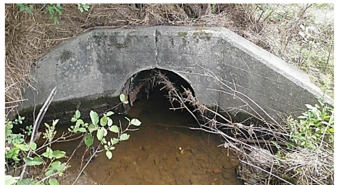
Figure 3-69: Examples of crossings with wingwalls and headwalls with square edges. (Image credit: NAACC)
