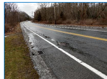
Figure D-5. Examples of good roadway photographs. The roadway photograph should show the condition of the roadway directly over the crossing and include any notable markers that would help locate the crossing in the future.
