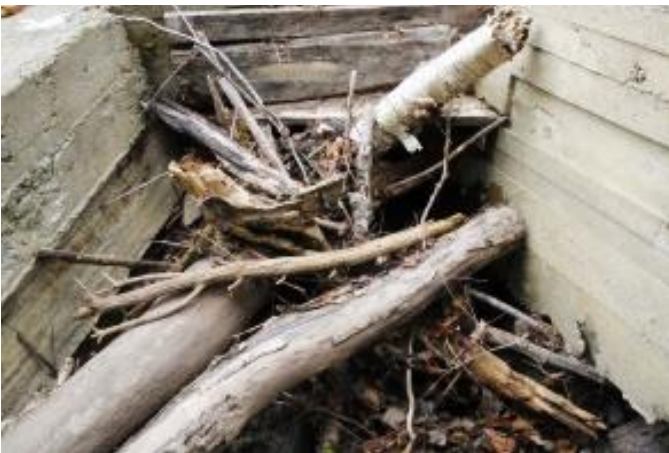
Figure 3-82: Example of a crossing with a clogged inlet. (Image credit: NAACC)
