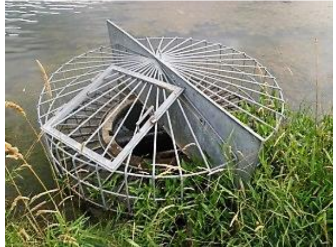
Figure 3-100: An example of multiple barriers, including fencing and a vertical drop. (Image credit: NAACC)
