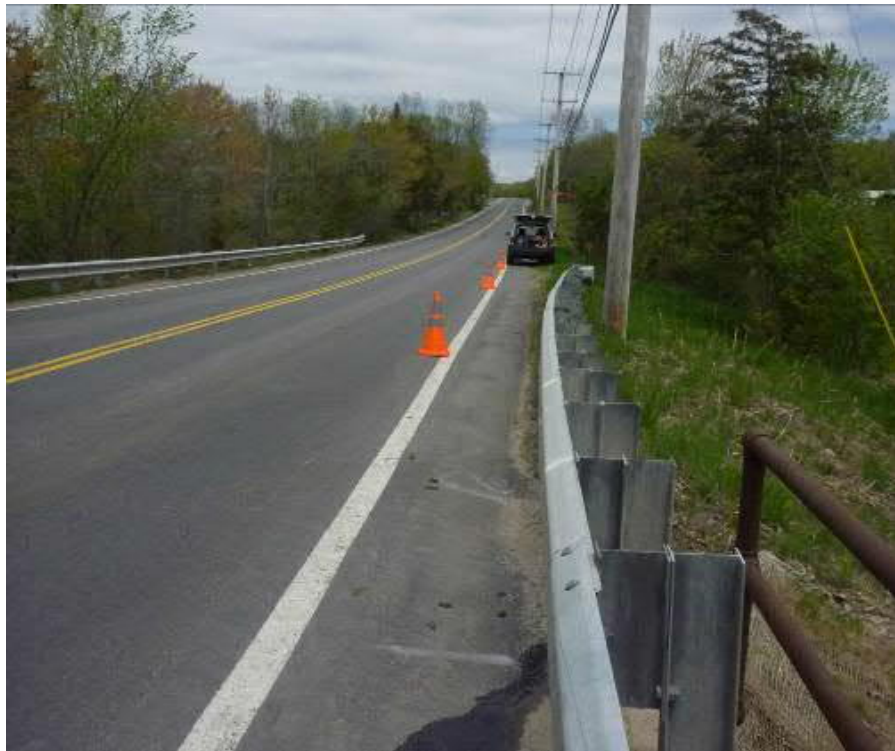
Figure 2. Cones set up on relatively high speed state route. Travel lanes are not blocked, and work will be less than one hour.
