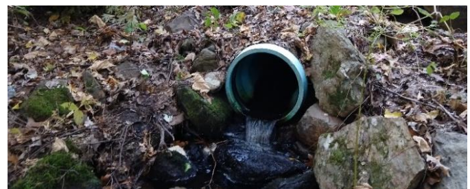
Figure 3-27: Material – Fiberglass.
