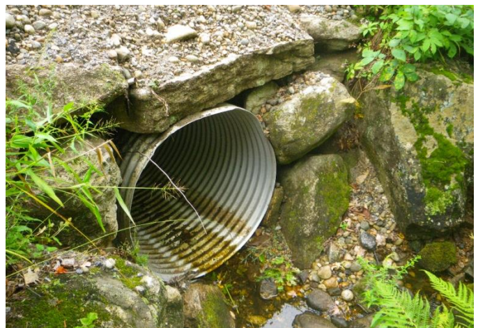
Figure 3-33: Material – Corrugated metal. (Image credit: NAACC)
