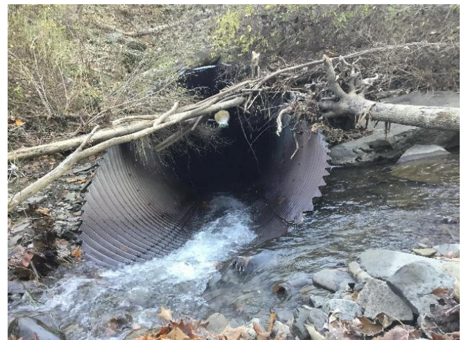
Figure 3-64: Examples of crossings with projecting inlets.
