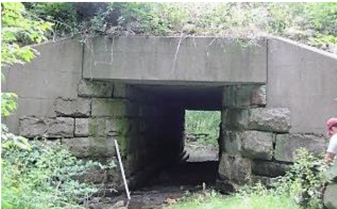
Figure 3-30: Material – Combination of stone and concrete. (Image credit: NAACC)
