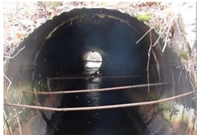
Figure 3-84: Examples of supports inside of road stream crossings. (Image credit: NAACC)
