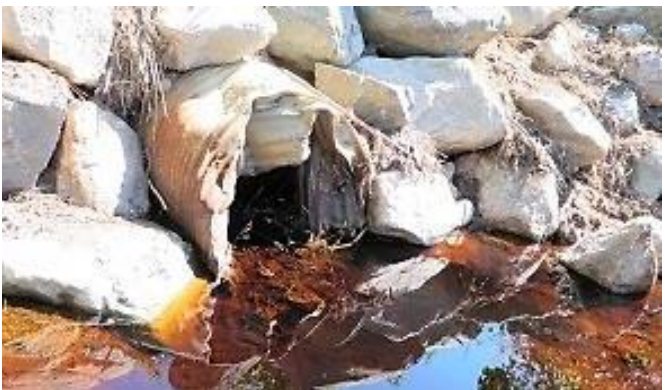
Figure 3-87: Deformation acting as physical barriers. (Image credit: NAACC)
